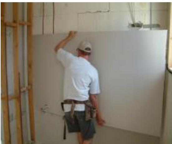
Wiring and plumbing is set into the polystyrene face, plasterboard is glued.
