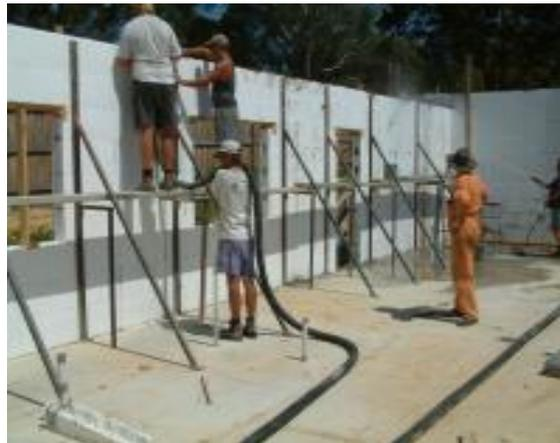
Formwork is braced and filled by pump.
